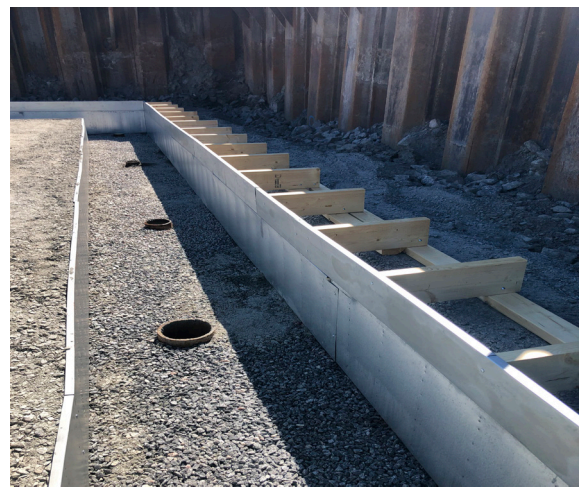
Edge Form with Extension Strip - Quick and Easy Height Adjustment On-Site
