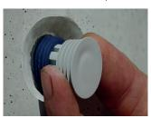
Hammer in the sealing plug with a single blow.
