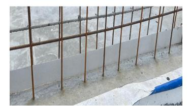
**3.** The installation depth (concrete cover) of the joint strip in the base slab should not be less than 3 cm after casting, to ensure proper encapsulation and long-term performance.
