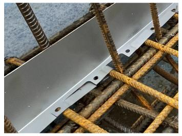
**2.** When overlapping, the joint strip must be overlapped by at least 10 cm, and the overlap should be reinforced with a joint strip clip (included with delivery). Each strip is clearly marked to indicate where the overlap
