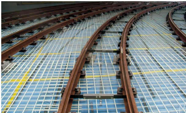
Floor slab railway depot Basel, Switzerland
