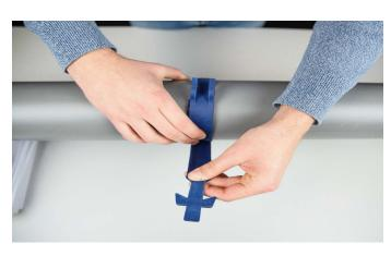
4. Verify that the HyDra Pipe Strap is securely fastened before starting the concrete pour.
